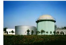
The project is a 300 cubic meters digester facility which is suitable for the treatment of manure of more than 12000 pigs and agriculture residues. The biogas is provided to local residents for cooking, shower and heating.
